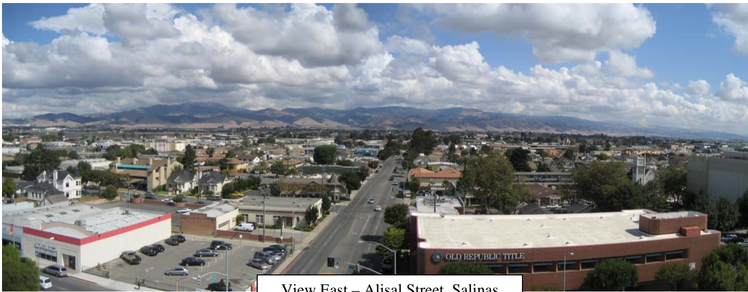
View East – Alisal Street. Salinas
